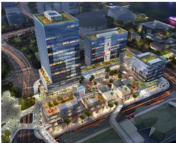
Mango West Bund Plaza, China
