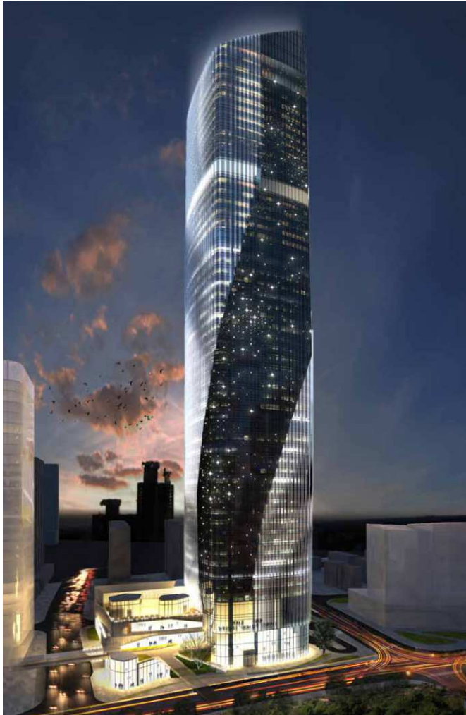
Ningbo New World, Ningbo, China
